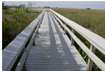
Figure 1. Boardwalk made from wood plastic composites in Everglades National Park in Florida
